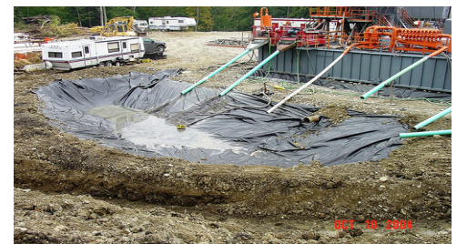
A waste pond is man made; it is used to dispose of contaminated waters created as a result of natural gas and other types of drilling.
